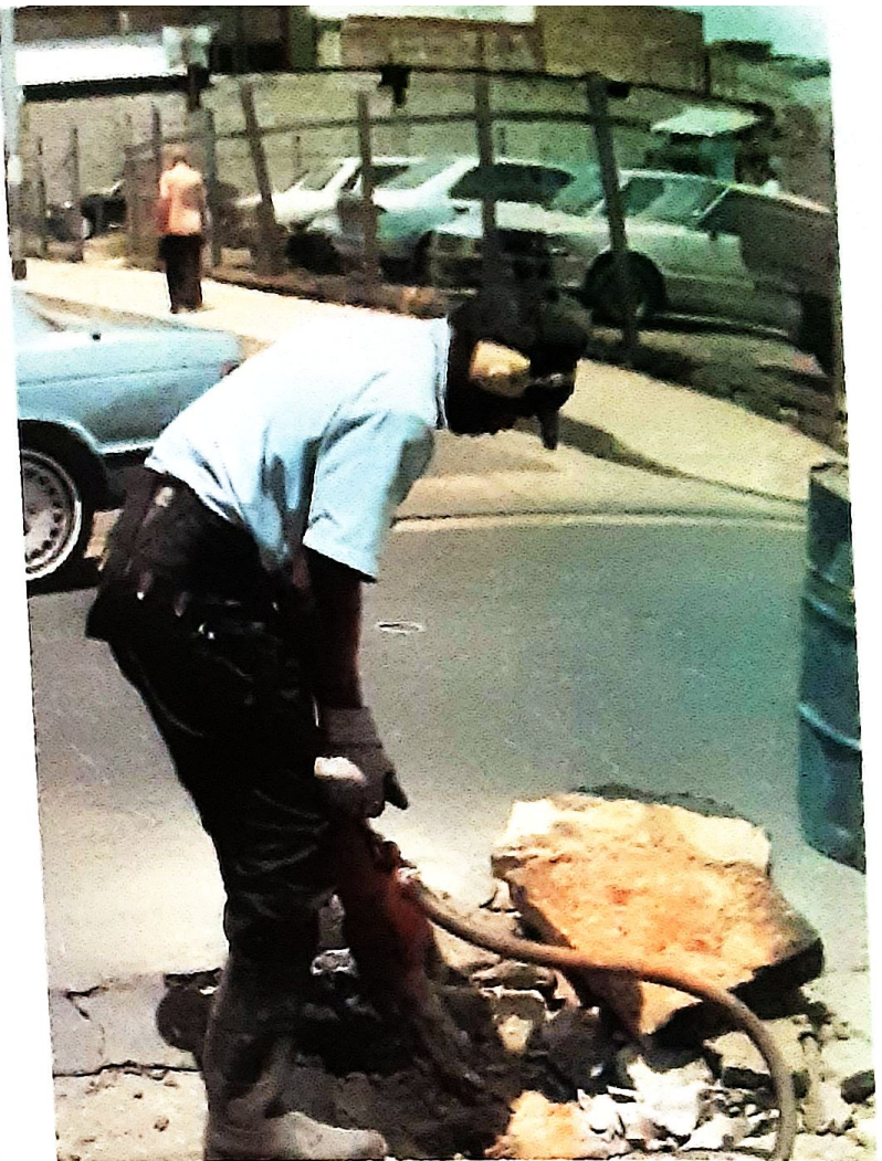
A worker wearing earmuffs to protect himself from the noise of the jackhammer
